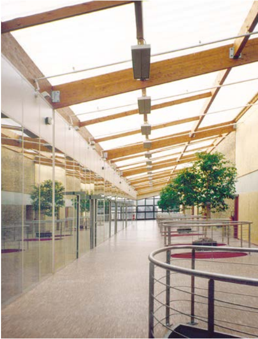
Corridors can be difficult to heat, but ceiling mounted EZ100 give off heat just where it is needed.
